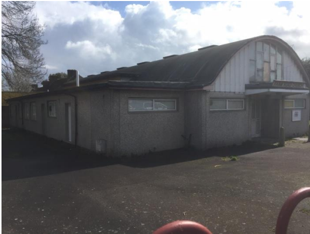
Canons Leisure Centre (22 Units)
